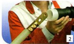
2 Place the 3M™ Cold Shrink termination body over the cable end and position at the correct point on the cable
