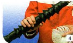
4 Once the inner core has been fully removed, the termination installation is complete!
