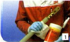
1 Prepare the cable as normal and clean with 3M™ Cable Wipes
